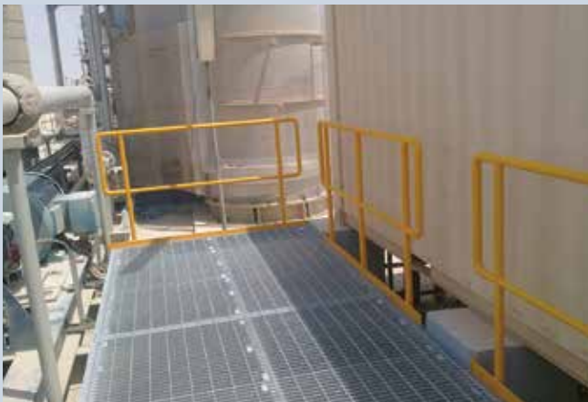
ACCESS PLATFORM / WALKWAY
